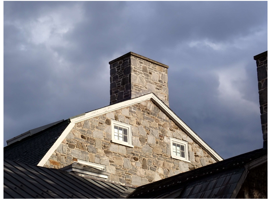
14. West elevation of main block, chimney detail, view southeast
