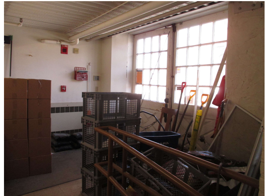
56. Lower level, service entrance vestibule, view northeast
