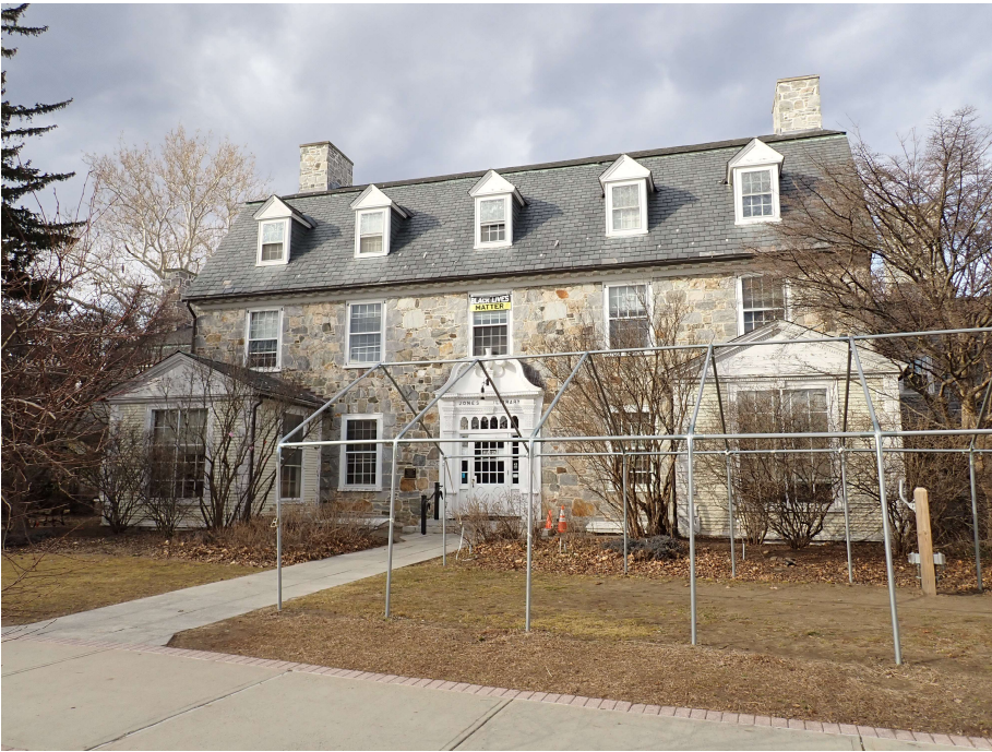
1. South elevation, view north
