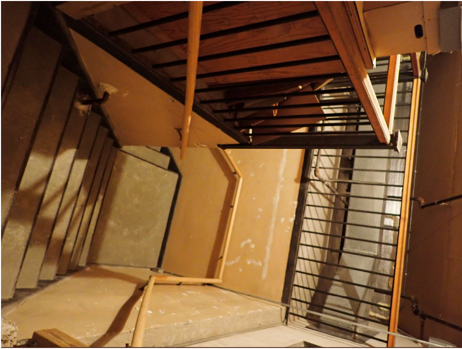
165. Attic level, main stair, view south
