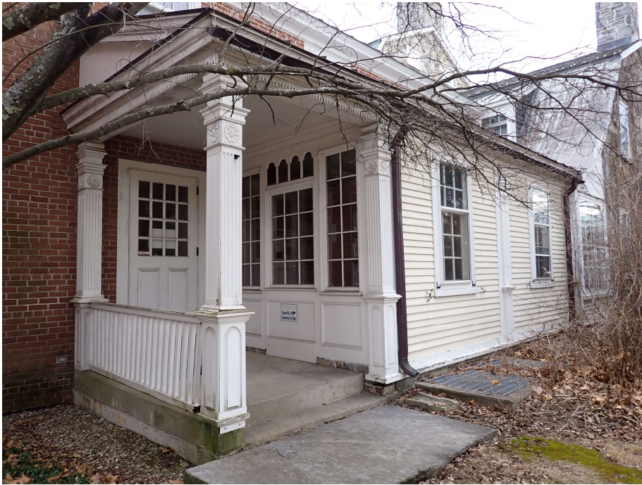
13. West elevation, secondary entrance, view southeast
