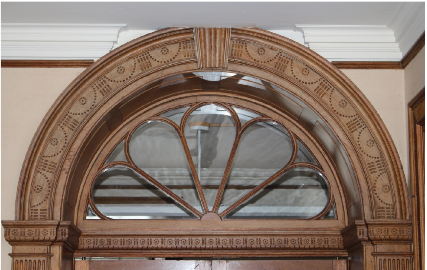
Fig. 22 Second floor, main stair hall. Close-up of the architrave showing the level of detail employed in its design. Note the carved keystone and the punch and gouge work used on the flats and the transom light. The paneled jambs of the arch are an added delight.
