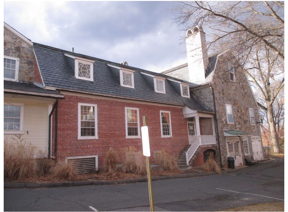
26. East elevation, view northwest
