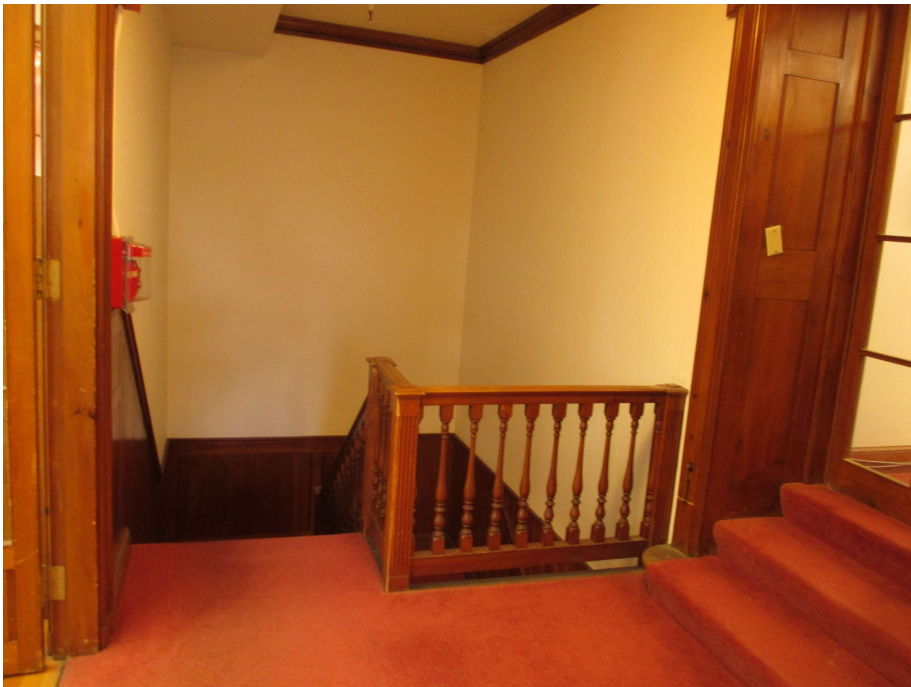
127. Second floor, southwest stair, view northeast
