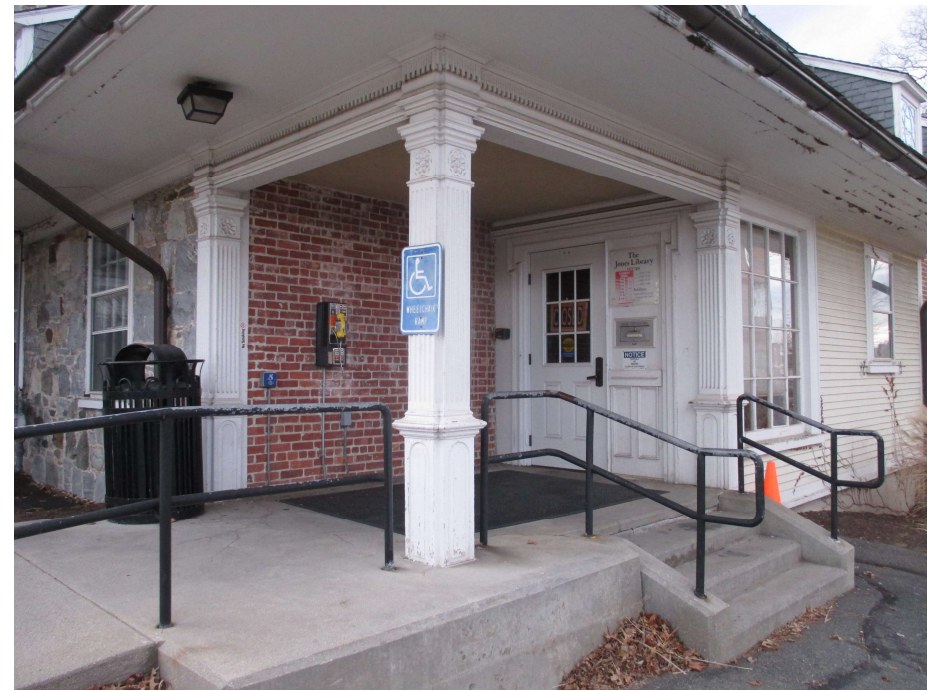
6. East elevation, primary active entrance, view northwest
