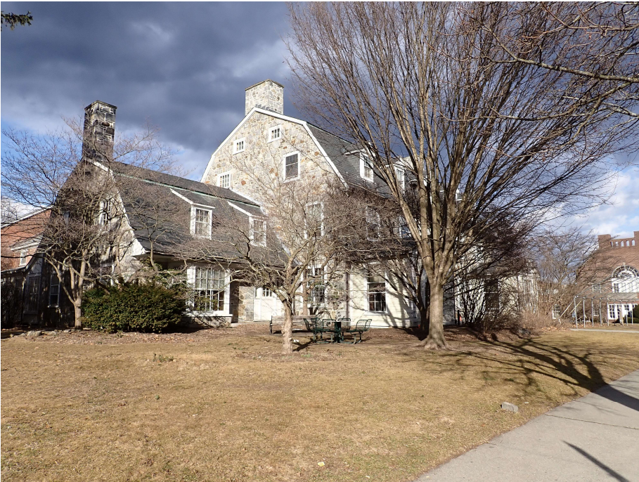
3. West elevation (left) and south elevation (right), view northeast
