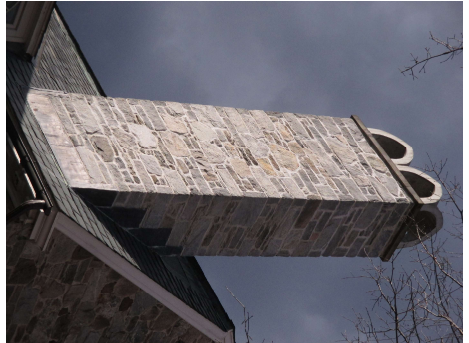
28. East elevation, chimney detail, view northwest
