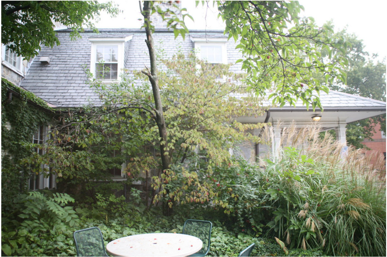
Fig. 50 East entry. The building is hidden behind a variety of different plantings that range in size and type. Vines should not be allowed to grow on wood surfaces. Large deciduous trees should be removed and kept well away from the perimeter of the building.
