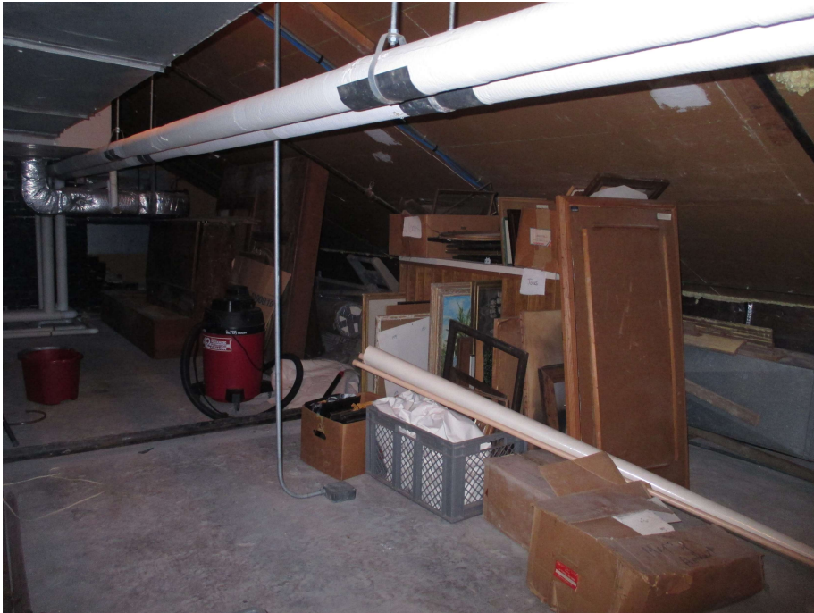
167. Attic level, view southeast
