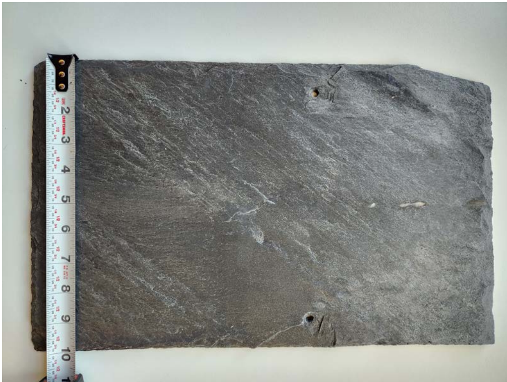
2. Salvaged historic Buckingham slate, typical condition
