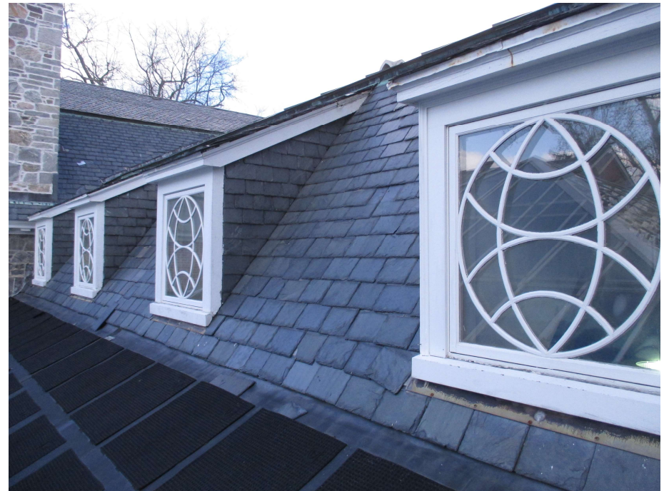
172. Roof level, view northeast
