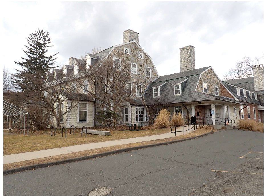
2. South elevation (left) and east elevation (right), view northwest
