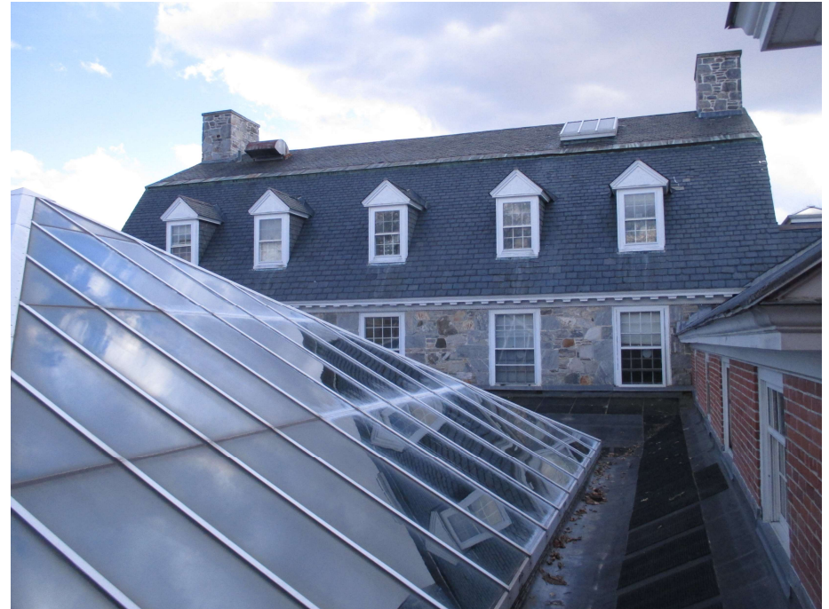
168. Roof level, view south
