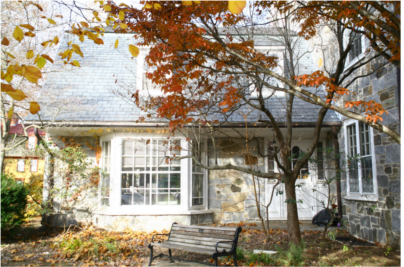
Fig. 8 West wing. The door here originally provided access directly into the children's stacks and reading room. This entry is no longer used. The door here is very similar to the doors that were located at the east entry prior to being converted into a universally accessible entry.
