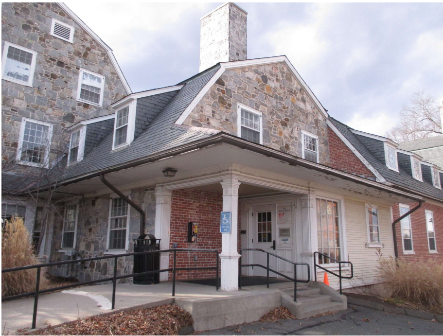
5. South elevation (left) and east elevation (right) of east wing and primary active entrance, view northwest
