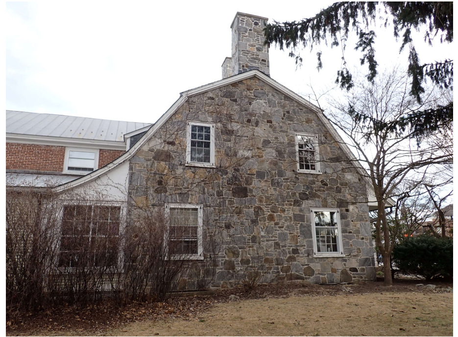
10. West elevation of west wing, view east
