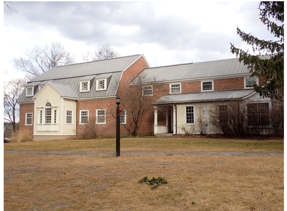
12. West elevation, 1990s additions, view northeast
