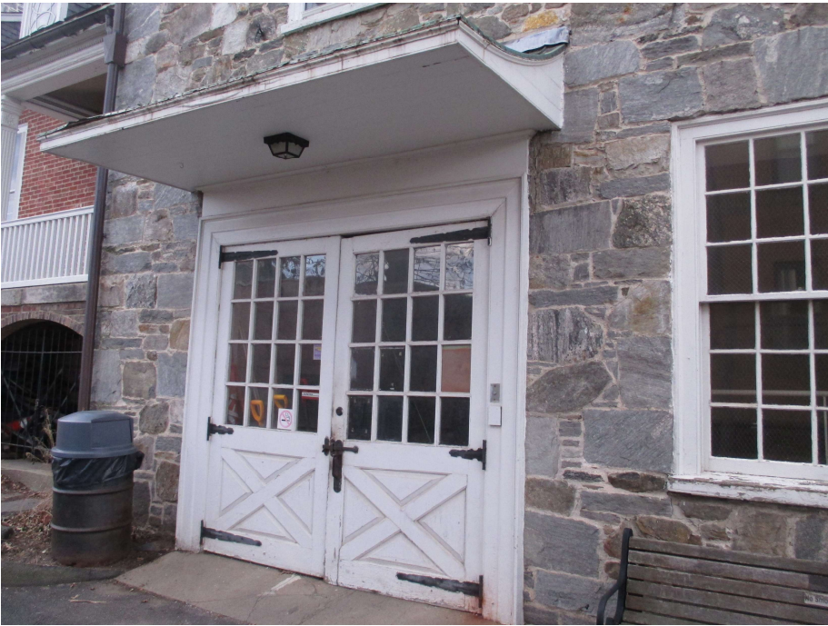
29. East elevation, ground level entrance, view southwest
