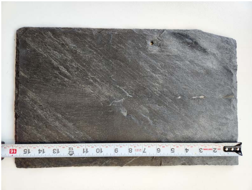
3. Salvaged historic Buckingham slate, typical condition
