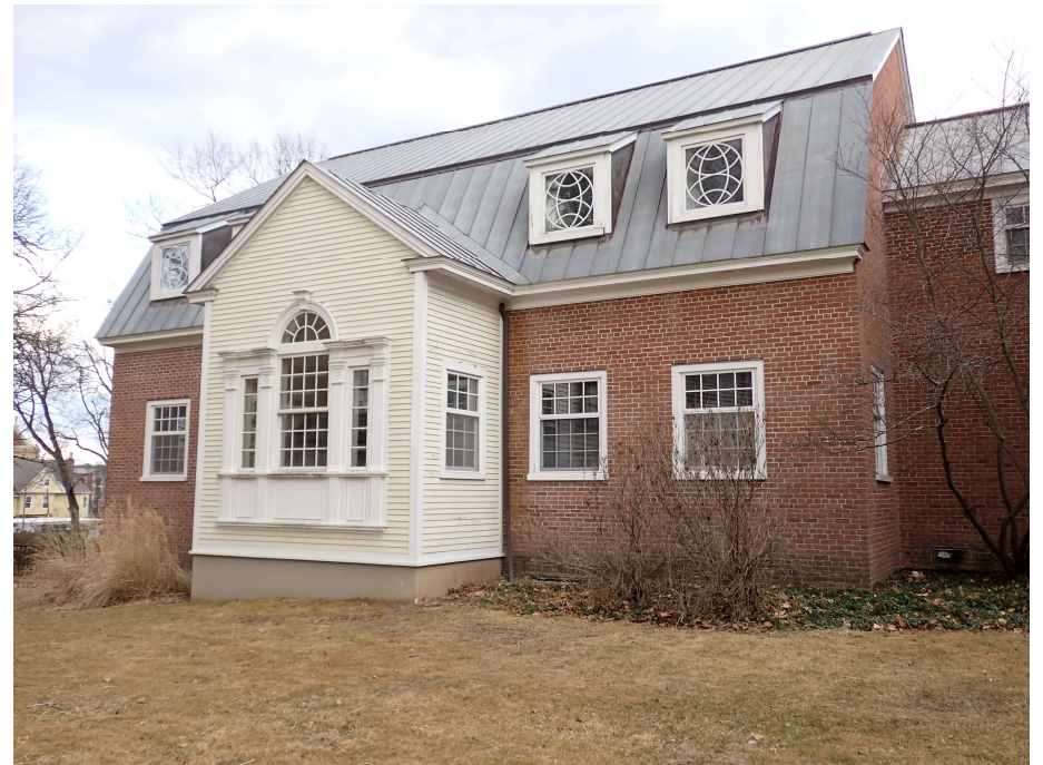
16. West elevation, view northeast
