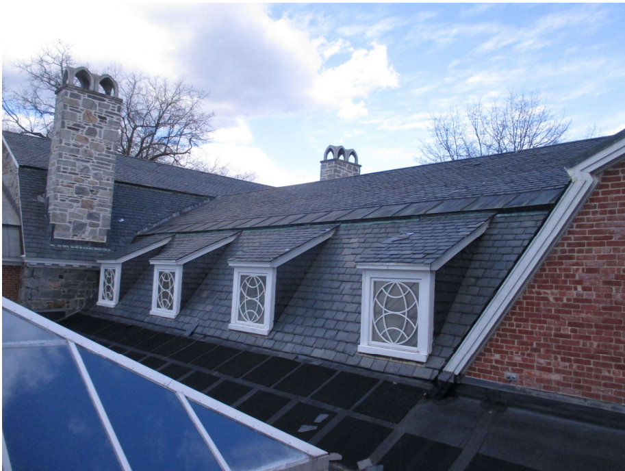
171. Roof level, view northeast
